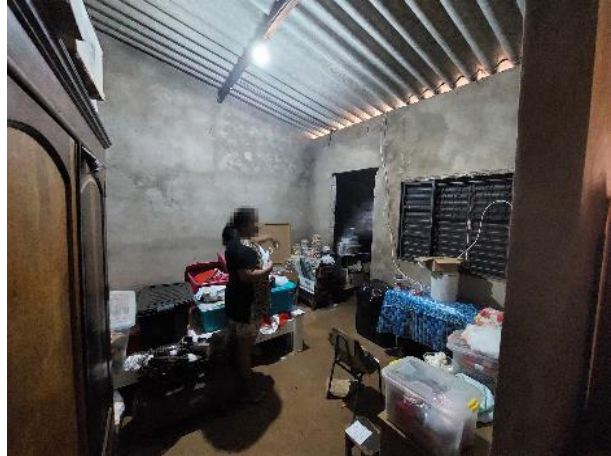
Figure 7 – Use of fiber-cement roofing without ceiling.
