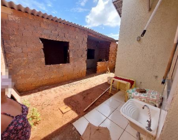
Figure 6 – Use of ceramic blocks in expansions.
