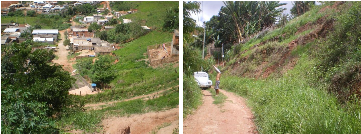
Figure 10 - Slope where the PMT-07 test was performed.
