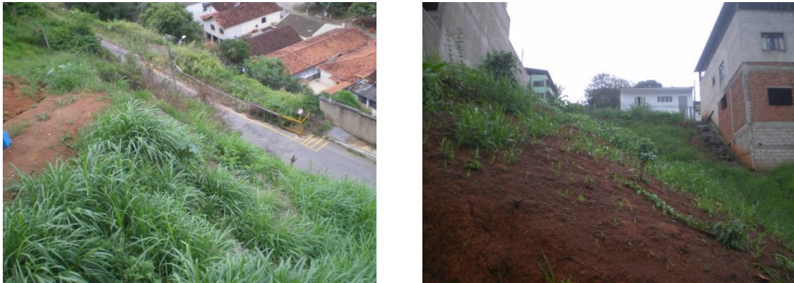
Figure 12 - Slope where the PMT-08 test was performed.
